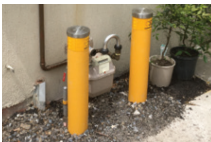
Compliant meter with bollards installed
