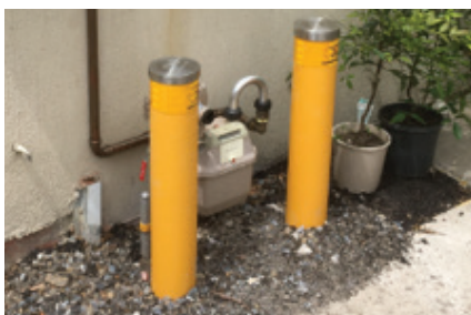
Compliant meter with bollards installed
