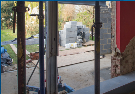
Site is not acceptable
