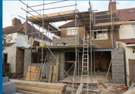
Site is not acceptable
